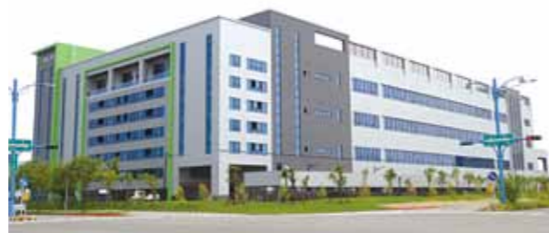
Siding (metallic composite panel) of Mildex Optical Inc. in Kaohsiung adopts Yieh Phui Crystallite Silky Pre-Painted Steel Sheets .
