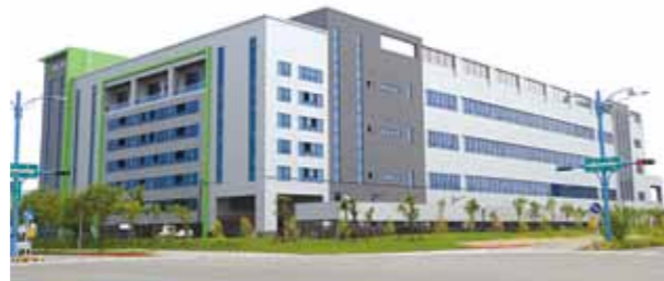
Siding (metallic composite panel) of Mildex Optical Inc. in Kaohsiung adopts Yieh Phui Crystallite Silky Pre-Painted Steel Sheets .
